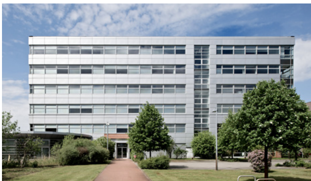
Berlin, Büro, Archiv, Refurbishment Bestand, 125 Mio. Euro
